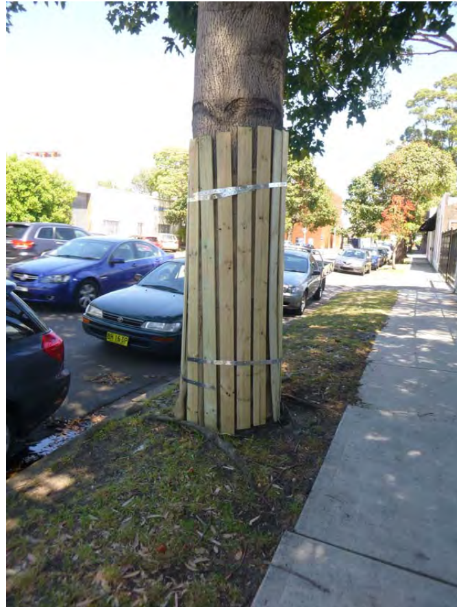
Figure 2.27 - An example of the minimum tree protection that would be required around an existing street tree while work is undertaken on an adjoining property (Photo: Arterra)
