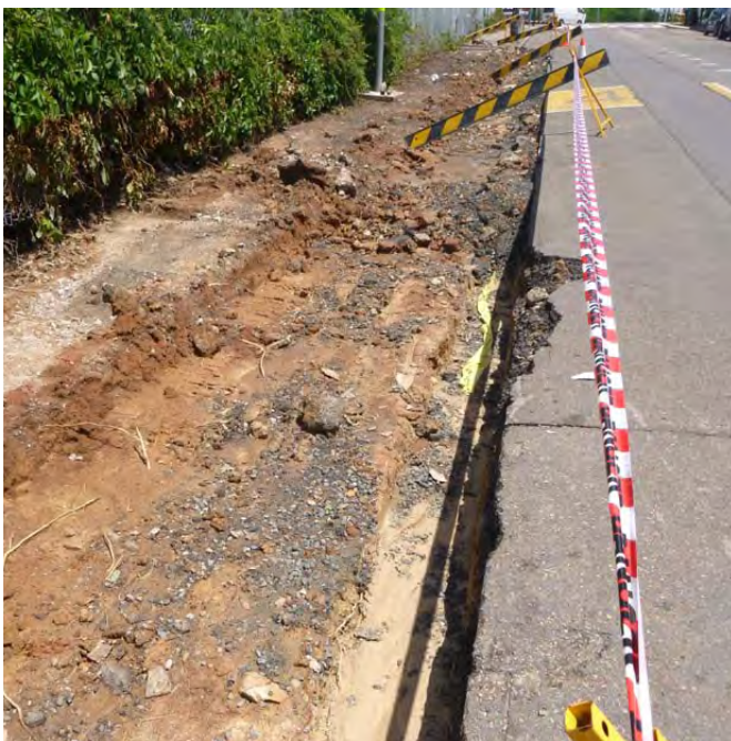
Figure 1.22 Hennessey St, Croydon - relatively good clay based soils dominate much of the area. These are easily compacted but have good water holding capacity and depth for tree establishment. (Photo: Arterra)
