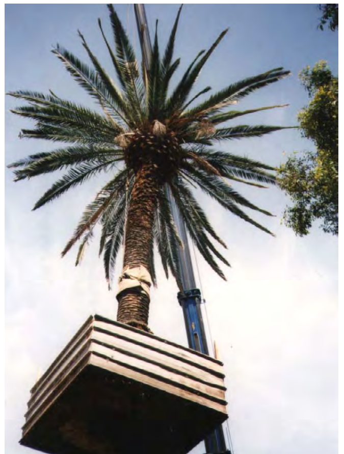
Figure 2.32 - Transplanting palms - boxed and craned (Photo-Arterra)
