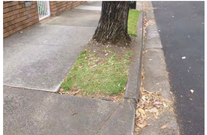
Figure 1.33 Cromwell St, Croydon South - example of narrow grass verge (Photo - Arterra)
