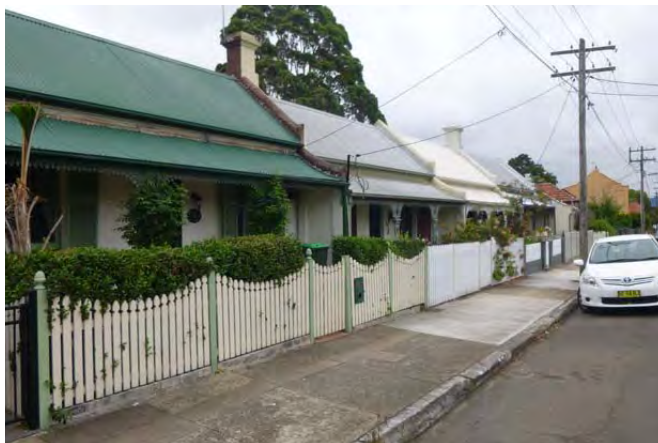
Figure 1.28 Lion St, Croydon - early workers style terraces (Photo - Arterra)
